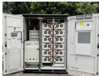
All-in-one battery cabinet 215kwh-100kw
